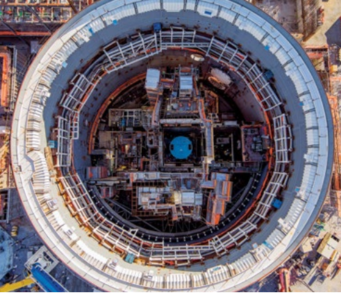
Bird's-eye view of Unit 3 nuclear island under construction at Georgia Power's Plant Vogtle, near Augusta, Georgia
